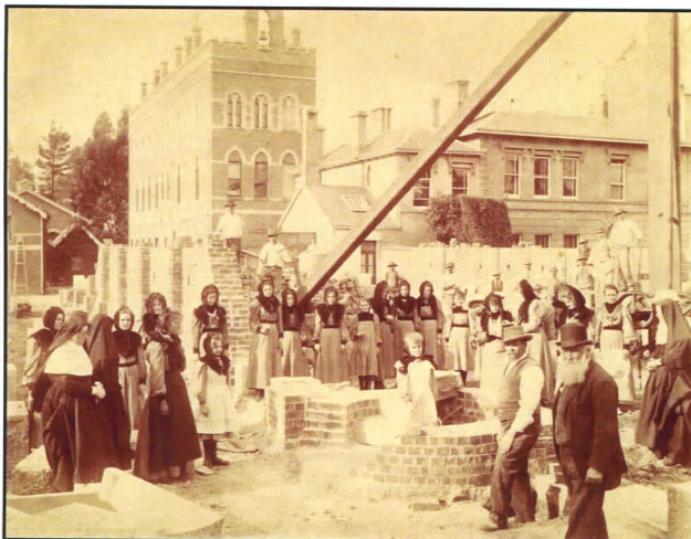
Above left: Laying foundation stone, 1899
